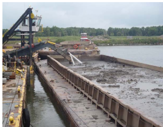
Small hydraulic dredge placing contaminated sediment into a disposal facility as part of the strategic dredging project in the River Raisin Area of Concern
