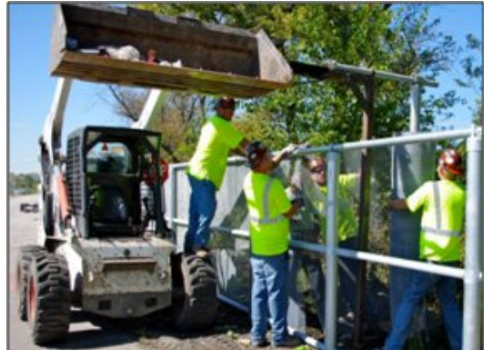
Workers installing the Des Plaines River invasive species prevention barrier
