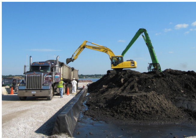
Contaminated sediment from the Division Street Outfall GLLA project (Muskegon Lake, Michigan) is processed and loaded for off-site transport to a disposal facility
