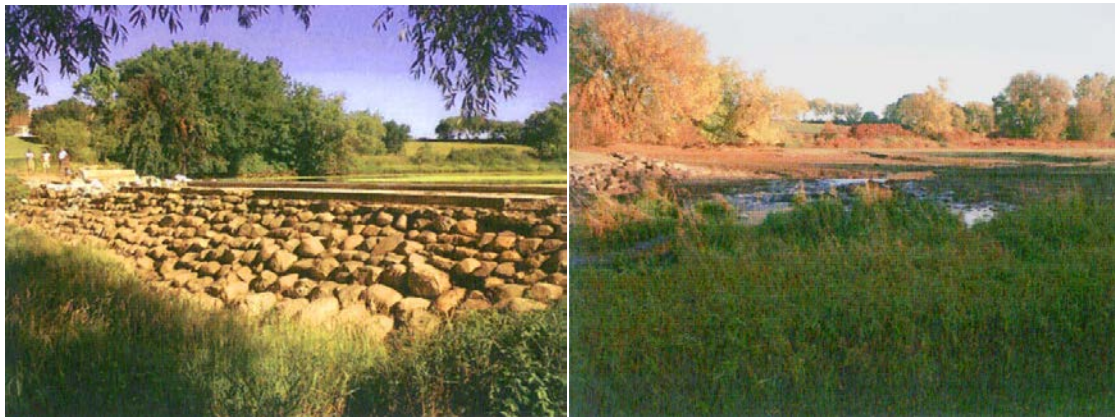
Images of the Campbellsport dam site pre-removal (left) and post-removal (right)
