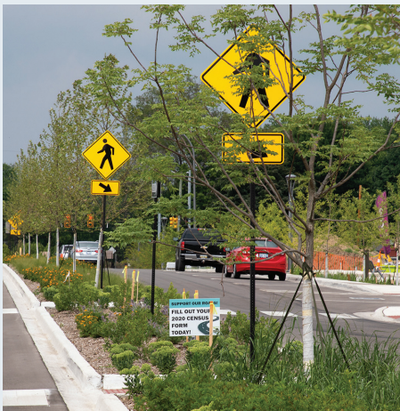
New green infrastructure development adds a rain garden to roadway to mitigate flooding. Photo Credit: Jon Clark, SEMCOG
