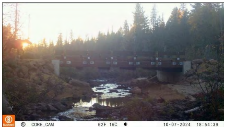
After: New bridge at Hockamin Creek Ramstad crossing (note moose crossing on the left!). Image: Jeff Jaspersen, MPCA
