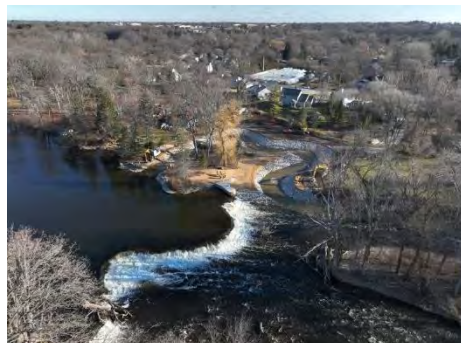
An aerial view of the Milwaukee River at Kletzsch Dam with the newly opened fish passageway. Image: Milwaukee Metropolitan Sewerage District
