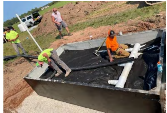
Installation of the water control structure for the Phosphorus Removal System at Kinnard Farms. Image: NRCS
