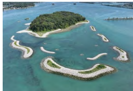
Aerial image of the completed restoration work at Sugar Island in summer 2024. Image: NOAA
