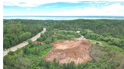
Aerial view during construction at Hartley Park. Image Minnesota Pollution Control Agency
