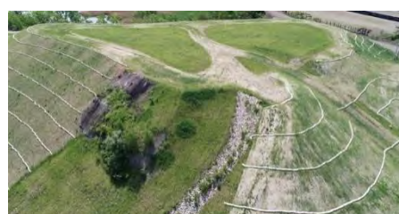
An aerial view of post-construction restoration of steel slag and steel mill waste areas, at the beginning of the first growing season. Image: Coldwater Consulting
