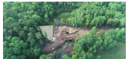
Aerial view: removing the culvert and embankment (September 2023). Image: NOAA Fisheries
