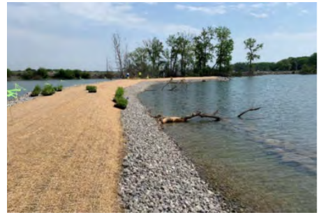
Image depicts barrier shoal islands constructed and planted with native vegetation as part of habitat restoration work in Hennepin Marsh. Image: NOAA
