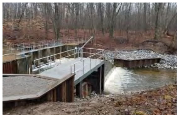
The permanent $1.67 million sea lamprey trap on the East Branch Au Gres River. Image: USACE
