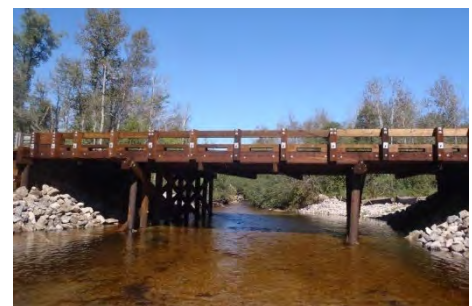
Maple River road crossing constructed using GLRI funding. Image: USFWS
